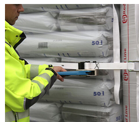
7. Secure the horizontal straps with a ladder buckle. Tension the horizontal straps with a tensioner.
